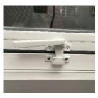
STEP 1: When the locks are straight, they are in the LOCKED position
