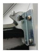
Catching the peg on the top swoop allows it to open to a 90-degree angle. To do this you will have to lift the sash all of the way up to be able to manipulate it into place. Let
