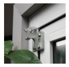
**STEP 3:** When the window is unlocked, raise the bottom towards you. Put BOTH HANDS on either side of the sash and move the hinge hook and peg where the frame and sash meet (glass portion of the window)
