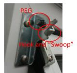
The peg slides back and you need to make sure the hook is secure. The bottom swoop allows it to open at a 30-degree angle. Make sure both sides have the hardware in the same position before letting go of the sash.
