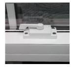
STEP 1: When the locks are to the left, they are in the LOCKED position
