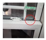
STEP 4: Locate the thumb buttons on either side of the locks.
