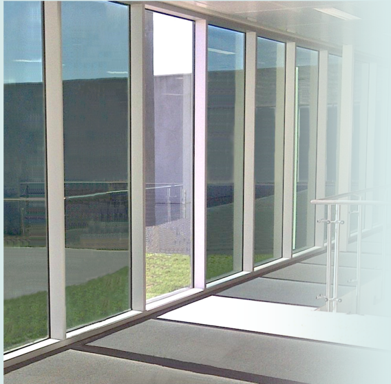
In the windows above there is one traditional window in between Suntuitive windows. The Suntuitive windows have tinted down to balance the brutal glare and heat that the traditional window is letting in.
