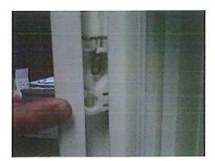
7. The sash can now be re-installed by angling the sash back into the frame and setting the pivot bars into the shoes.
