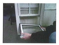
4. Completely remove sash by lifting other corner of sash up:
