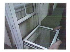
3. Angle one corner of the sash out of the frame:
