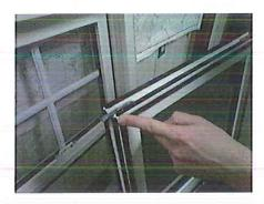
6. It needs to go back into the "shoe". There's a rectangular opening in the shoe that needs to be turned to an "up-and-down" position. Use a large flat head screw driver if this opening needs to be rotated to the position seen below:
