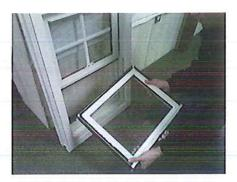
5. Notice the "pivot bar" located at bottom of sash:
