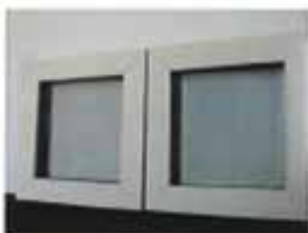
Darker Low-E reduces FREE energy from the sun (Polar Seal on left)
